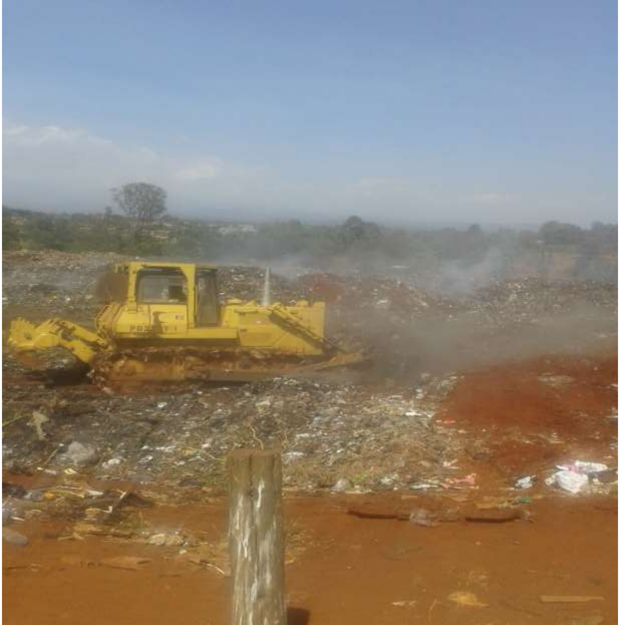
CLEARING OF THE DUMP SITE AT ASIAN QUARTER IN NYERI TOWN.
