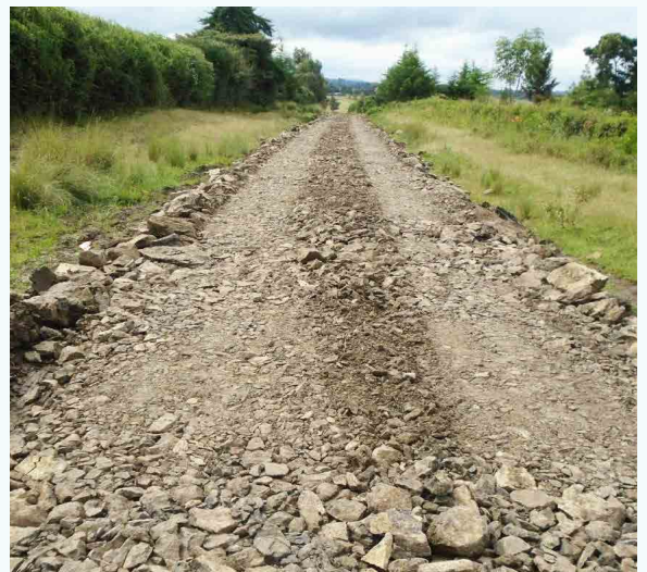
Upgrading of Villa road in Kabarú ward, Kieni East sub-county almost complete.
