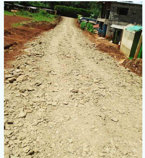
Upgrading of Game Rock Shopping Centre in Kiganjo / Mathari ward, Nyeri Central sub-county has commenced.
