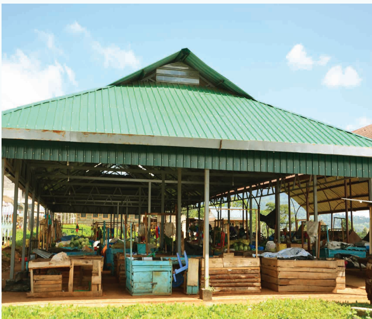
The new face of Kamakwa market in Kamakwa ward after roofing and cabro paving work. This has improved the working environment of the 100 traders who are conducting their businesses at the facility.
