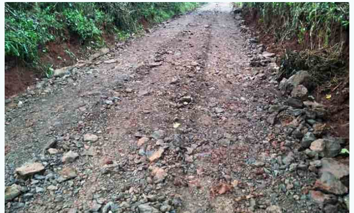
Upgrading of Gikoro road in Rugi Ward, Mukurwe-ini sub-county almost complete.
