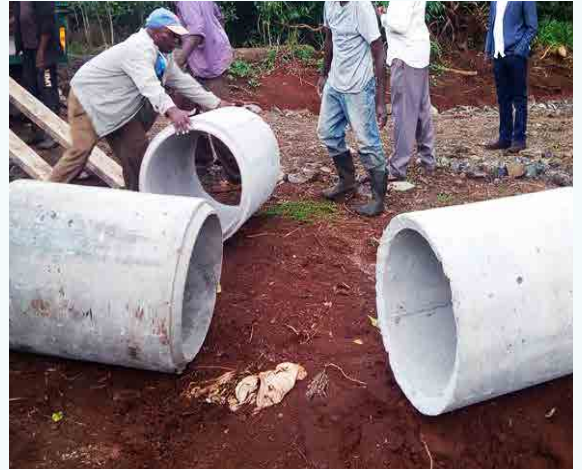
Process of improving drainage systems by installing culverts in Kirmukuyu ward, Mathira West has already kicked off.
