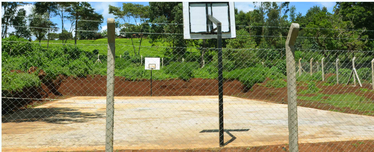
The new Kinunga Basketball court in Dedan Kimathi ward, Tetu sub-county. BELOW: Upgrading of Ngangarithi Primary School - Muthaiga Estate road, Kamakwa ward to bitumen standard on progress.
