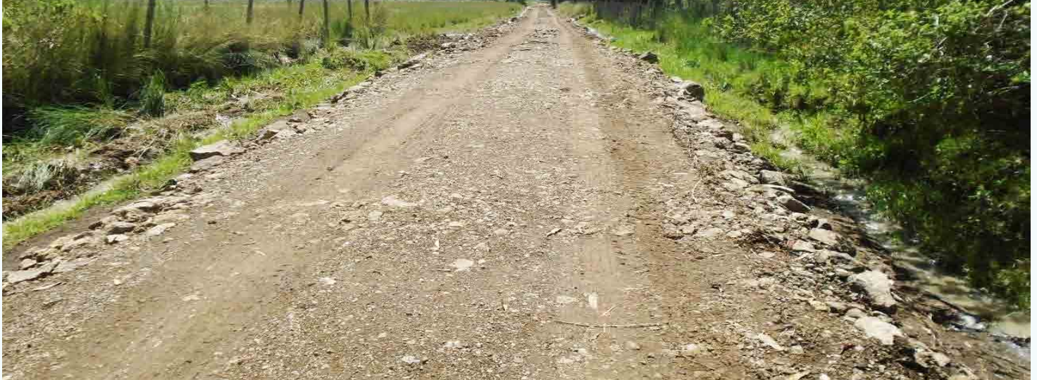
Recently upgraded Muthenya-Kihara Road in Naromoru/Kiamathaga ward, Kieni East sub-county. Culverts were also installed.
