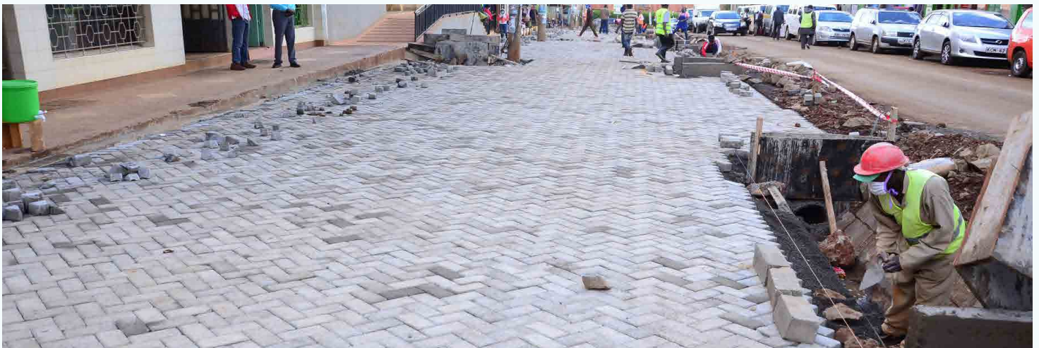
Upgrading of parking slots using cabro paving blocks along Gakere Road, Nyeri town in Rware ward on progress.
