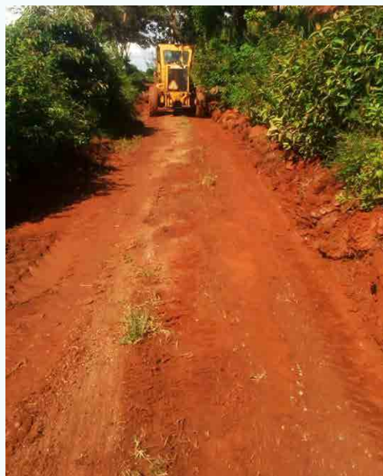
Progress of Gitumbi road upgrading in Mweru area, Rugi ward, Mukurwe-ini.
