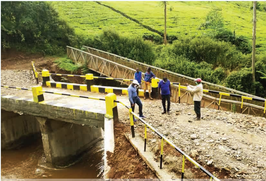
ABOVE: The new modern Matiriongo Bridge in Chinga ward, Othaya, which was last done in the 1960s, is now complete and operational. More photos of projects on page 2,3 & 5.
