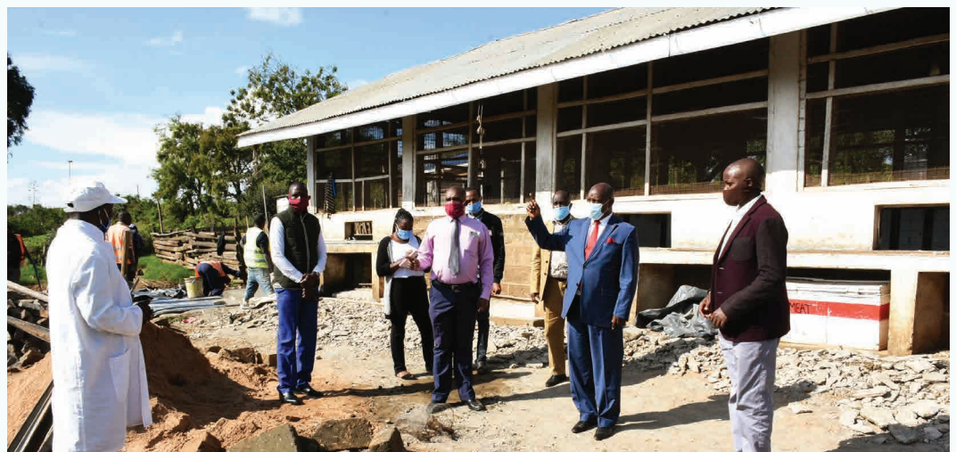
The governor (second right) inspecting the ongoing refurbishment of Mweiga slaughter house.
