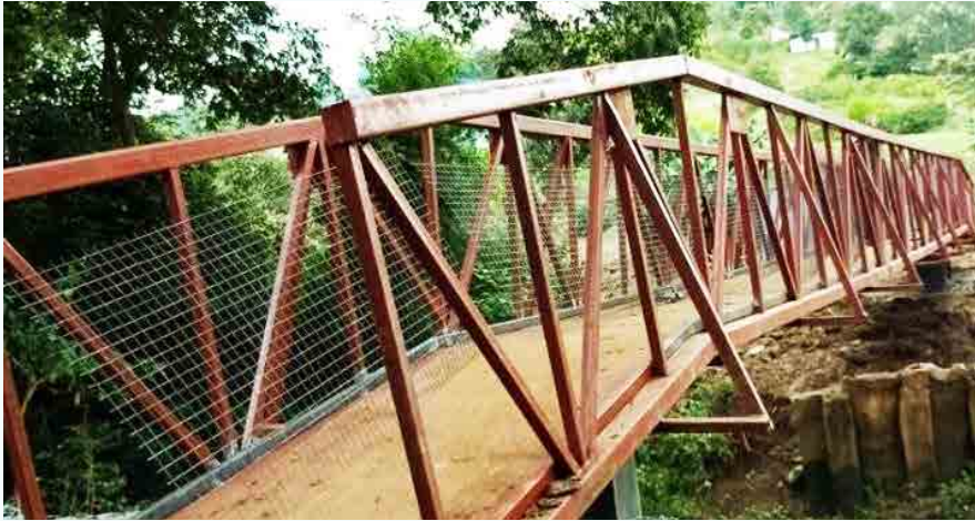
Ongoing Kiganjo/Gatei footbridge in Kiganjo/Mathari ward, Nyeri Central sub-county is almost complete. The footbridge will enable easy access of residents in the area.
