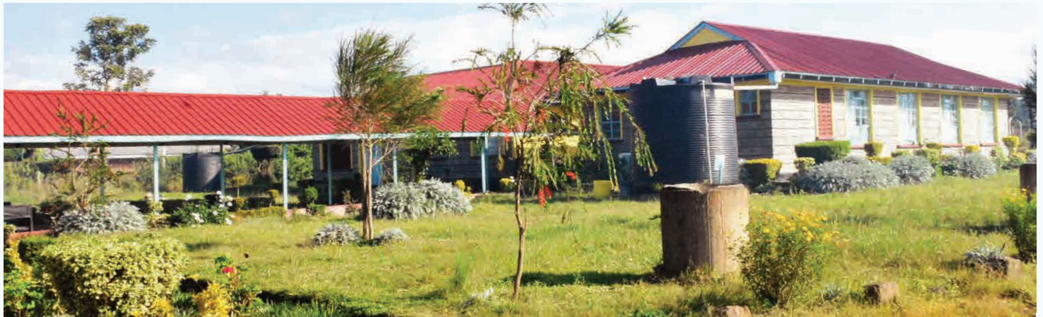
The newly refurbished Mweiga Health Centre in Mweiga ward, Kieni West sub-county by the County Government of Nyeri.
