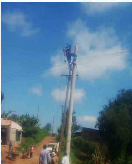
Installation of street lights at Gathagara, Kiang'onde, Thangathi Poly and Mbugwa (nuru center) in Mukurwe-ini Central ward.
