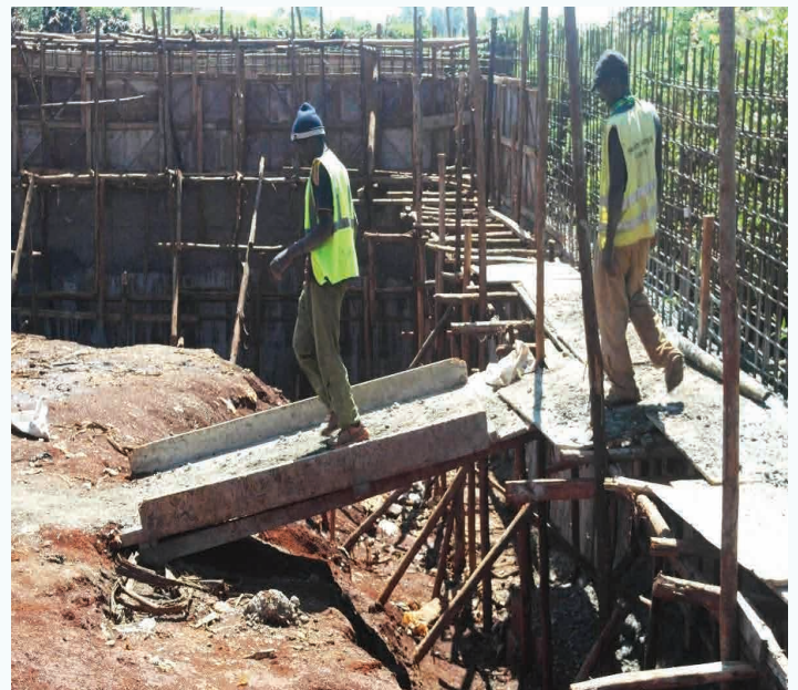
The construction of the retainer wall in the Nyeri Bus Termini is ongoing.
