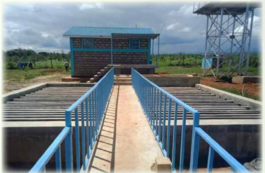
The County Government of Nyeri has constructed a water treatment plant at a cost of Kshs. 34 million in Kieni East sub county and Tana Water Works Development Agency (TWWDA) has financed a new water pipeline at a cost of Kshs. 10 million.
