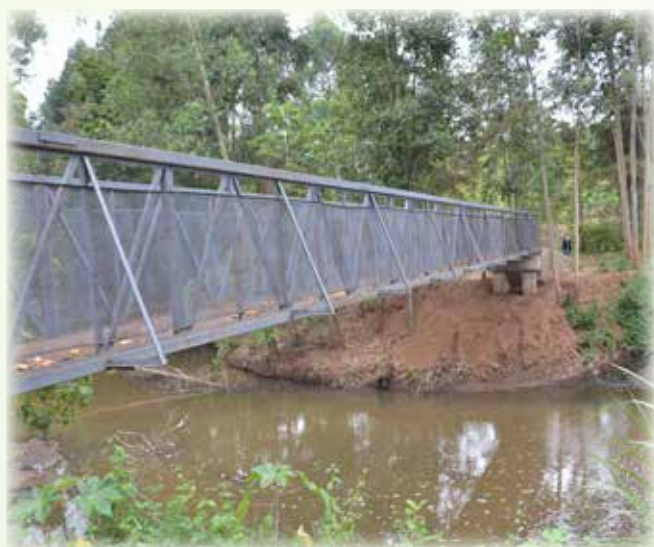
The new Kahiga - Kahira-ini footbridge in Kiganjo / Mathari ward.
