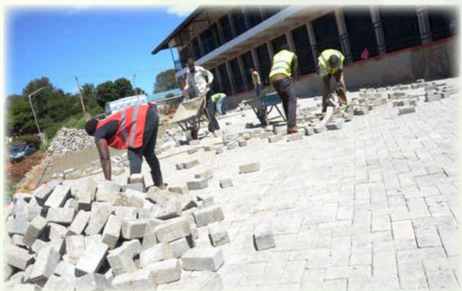
Workers upgrading the roads using cabro paving blocks within the ongoing Nyeri Main Bus Termini at Asian Quarters, Rware ward, Nyeri town.
