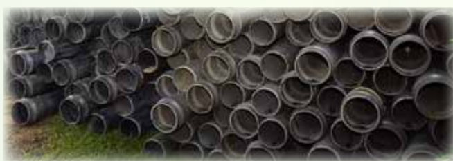
Water pipes for the ongoing Ihuririo Irrigation Water Project in Iria-ini Othaya ward.
