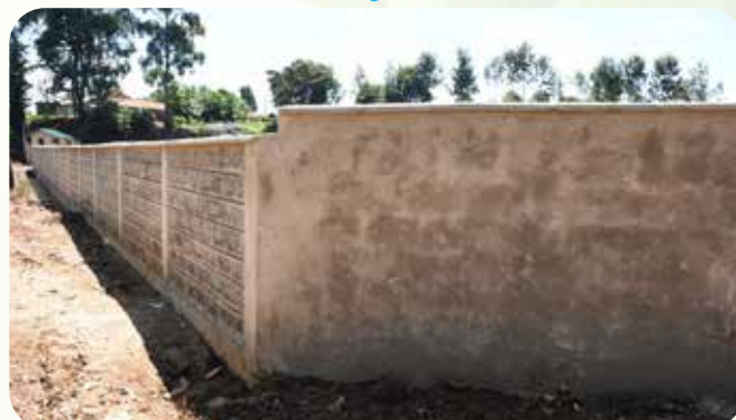
Newly erected perimeter wall at Gikeu dumpsite in Karima ward, Othaya.
