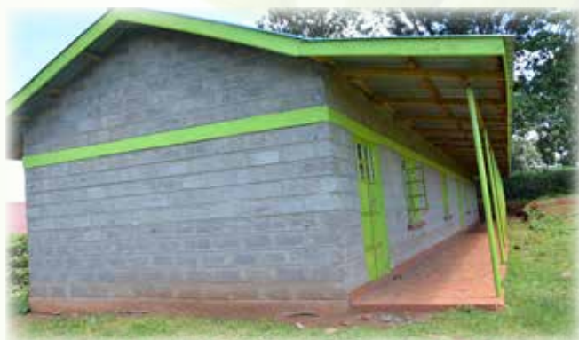
The new Kamuyu ECDE classrooms in Kamakwa ward, Nyeri Central sub county.
