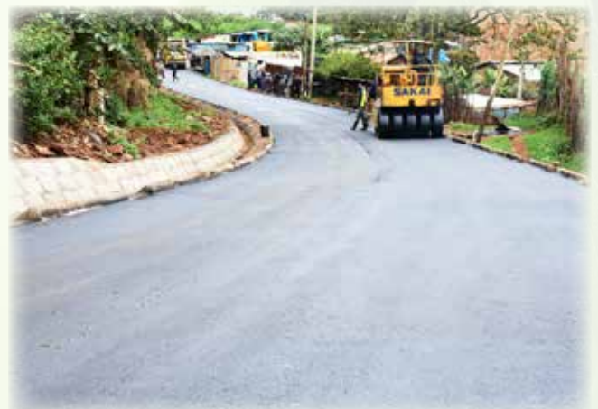
The newly tarmacked Library- Nyewasco road in Nyeri town.
