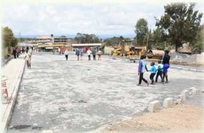
The new Mweiga Bus Park which was upgraded using cabro paving blocks.
