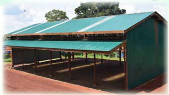
The ongoing construction of Mihuti market in Rugi ward, Mukurweini sub-county.
