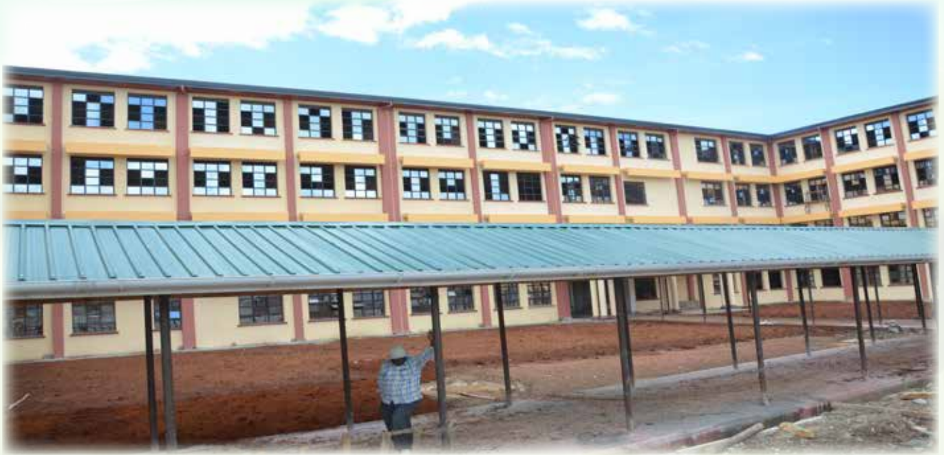
The ongoing progress of Naromoru Level 4 Hospital in Kieni East sub county.
