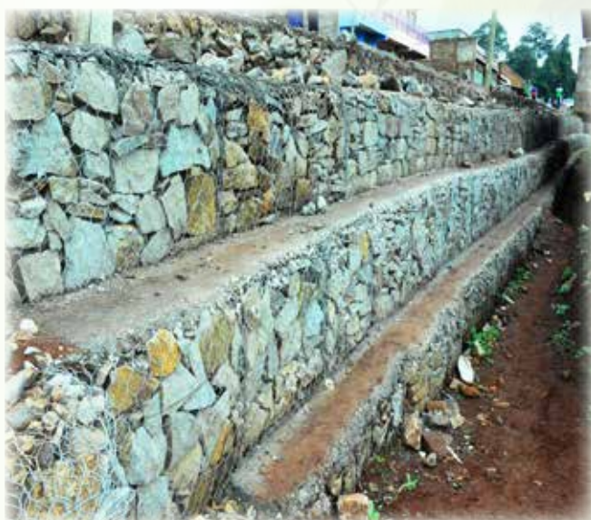
The second phase of Kianda road, Nyeri town upgrading to bitumen standard has kicked off.
