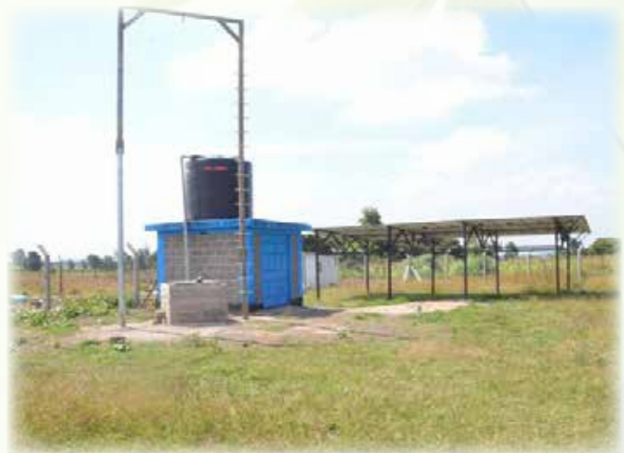
Biricha Borehole project in Mugunda ward, Kieni West sub county.
