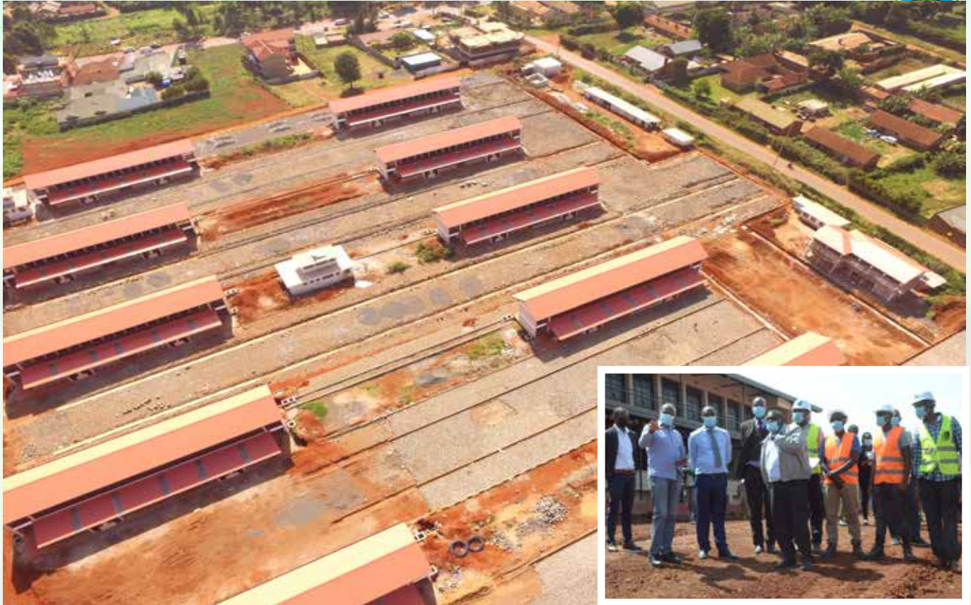
An aerial view of the upcoming Nyeri Main Bus Termini at Asian Quarters, Nyeri Town. INSET: A team from the Kenya Urban Support Programme (KUSP) during the monitoring and evaluation visit at Nyeri Main Bus Termini. They were accompanied by the Nyeri Municipal Board members and Lands CEC Dr. Kwai Wanjaria (3rd left).
