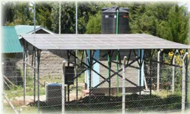
Solar powered Mapema borehole project in Kabaruu ward, Kieni East sub county.
