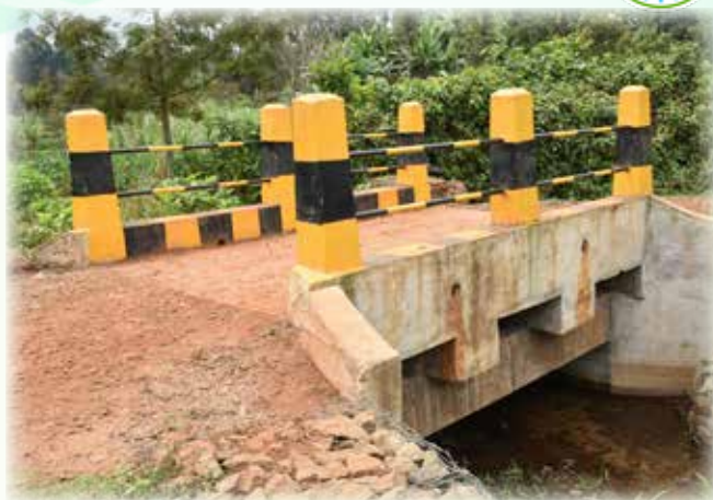
Kinyariti box culvert in Iria-ini ward, Mathira East sub-county.
