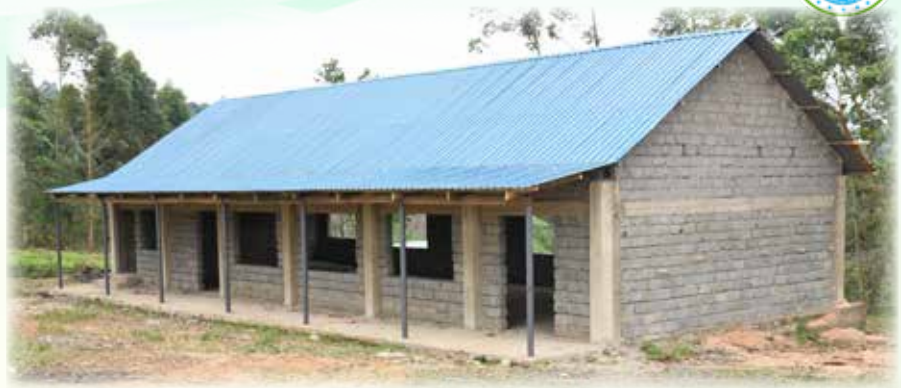
Progress of Kariki Social Hall in Iria-ini ward, Mathira East sub county.
