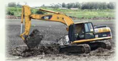
An excavator desilting Lusoi dam in Thegu River ward, Kieni East sub county.
