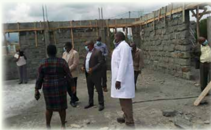
Ongoing construction of a new multi purpose hall at Nairutia Vocational Training Center in Mugunda ward, Kieni West sub county.
