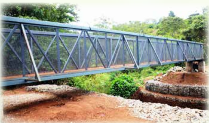
The new Kirichu Thagwanja footbridge in Kiganjo / Mathari ward.
