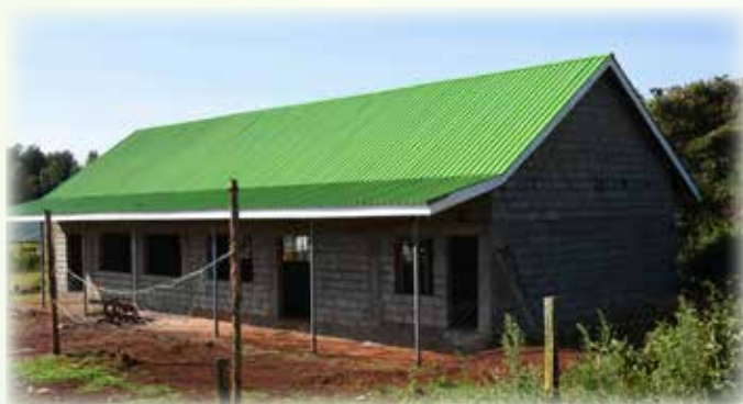
Progress of Muruguru Social Hall in Gatitu / Muruguru ward, Nyeri Central sub county.
