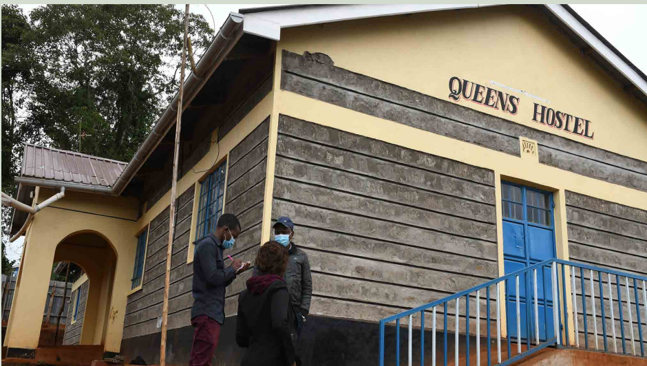
Queens Hostel at Karatina Vocational Training Centre in Karatina town, Mathira East sub county has been completed. The hostel had initially stalled due to lack of funds.
