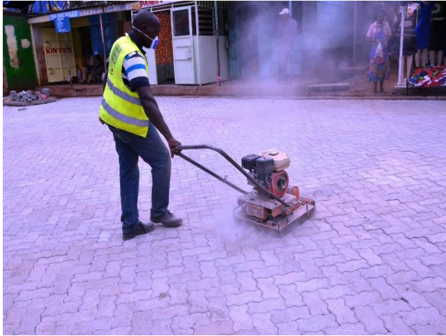
Upgrading of Kuku Lane to Cabro
