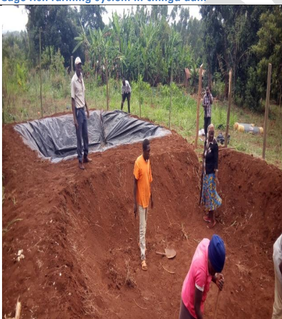
Fish Pond construction activity in Mukurweini Sub County
