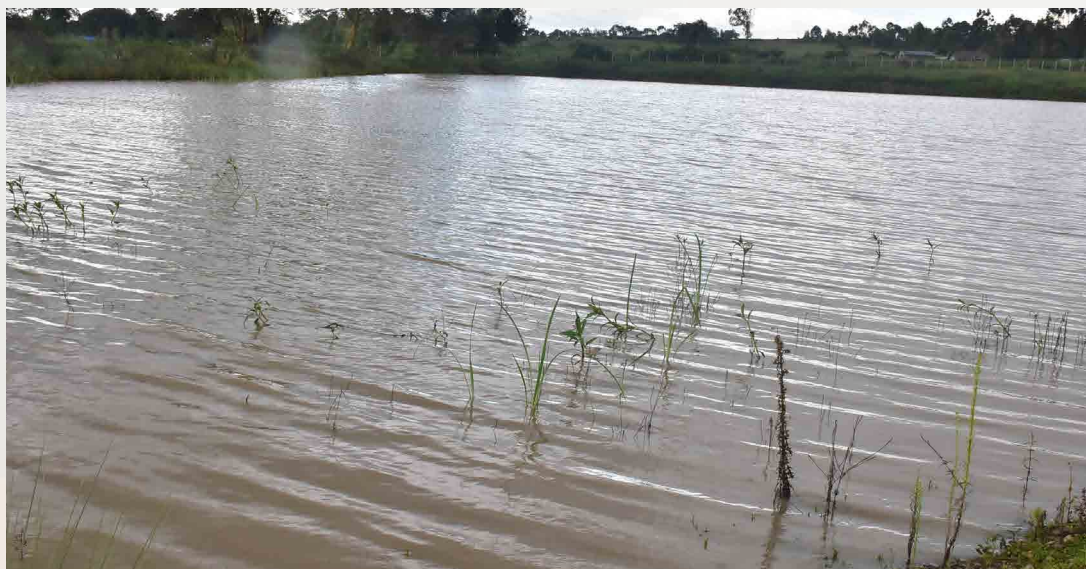
Lusoi Earth Dam in Kieni East sub-county which was rehabilitated and desilted through KCSAP. Upon its completion, it has benefitted over 800 members. (Below) Kiria Earth Dam in Watuka, Kieni West sub-county which has the capacity to hold water for irrigation for 90 days. Through KCSAP, it was rehabilitated, fitted with solar panels which pump water to a storage water tank which is then distributed to the beneficiaries.
