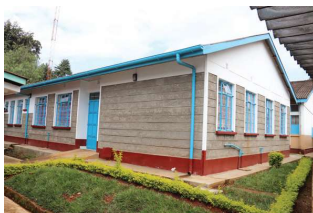
Newly Constructed New born unit at Karatina Sub County Hospital
