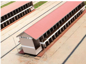
Newly Constructed Asian Quarters Transport Terminus
