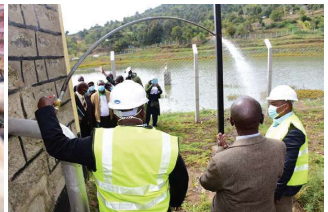
Commissioning of the rehabilitated Kiria Dam
