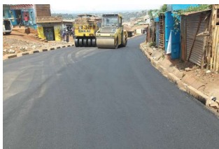
Tarmacking of Kianda road, Nyeri town
