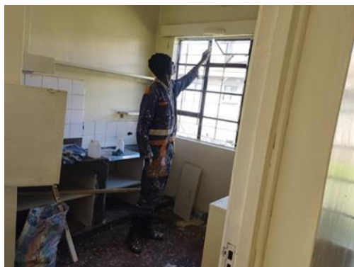
Renovation of county residential unit at Muthaiga estate
