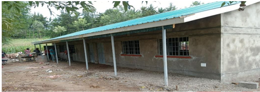
Renovated Kiriti ECDE twin classrooms
