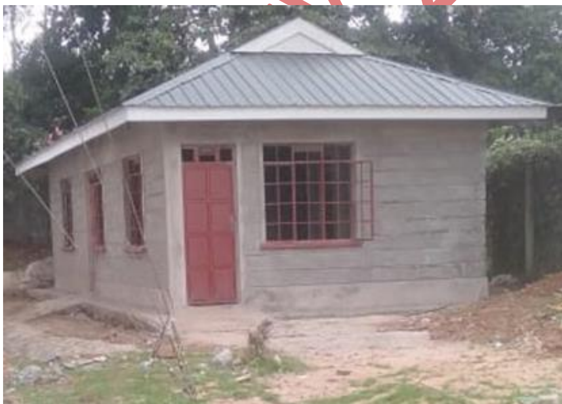
Construction of a sanitary facility at Karatina
