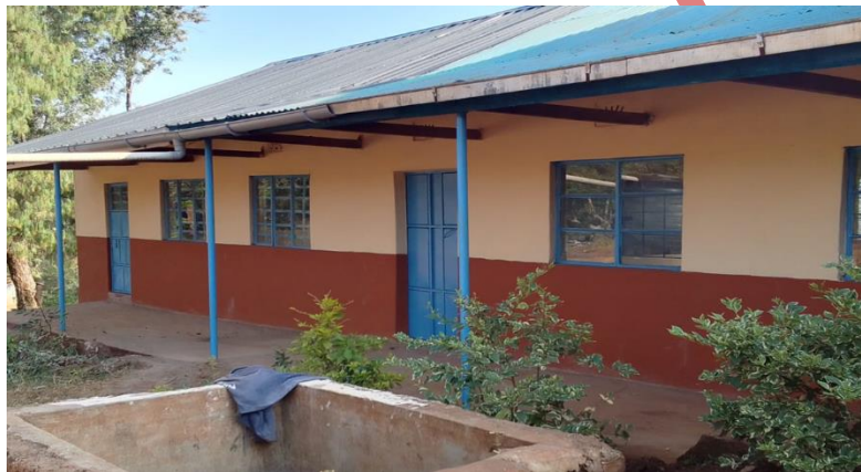
Renovated Karaba ECDE centre classrooms in Gikondi Ward
