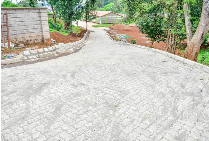
Cabro paving at Nyeri Cultural Centre
