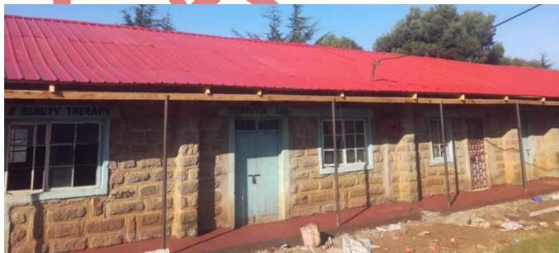
Renovated Watuka VTC Classrooms
