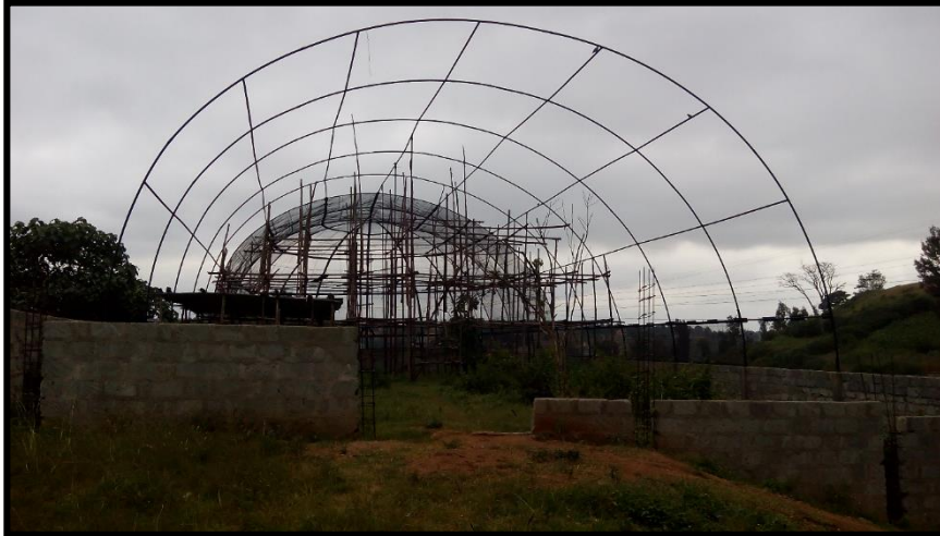
Figure 68: Cultural Center under Construction
