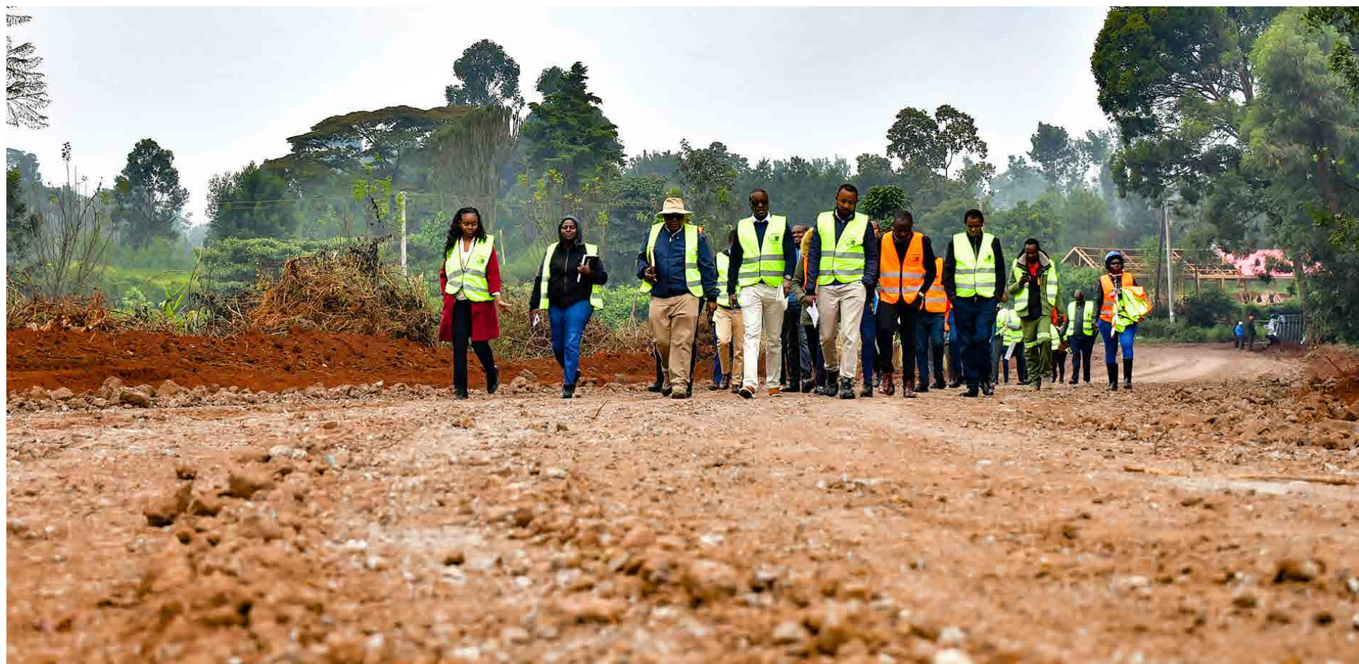
KISIP II team inspecting the ongoing informal settlements upgrading in Nyeri County.
