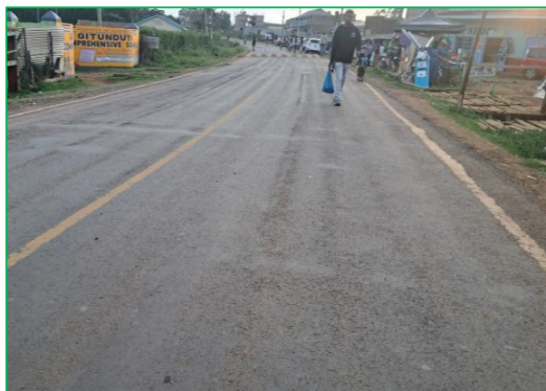
Karatina – Gaikuyu – Gitunduti Road (E602) (Tarmacked)
