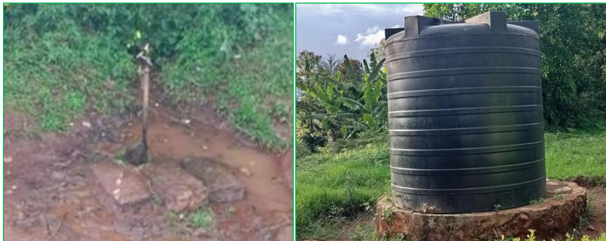
Plate 5: Water Supply and Storage Facilities
