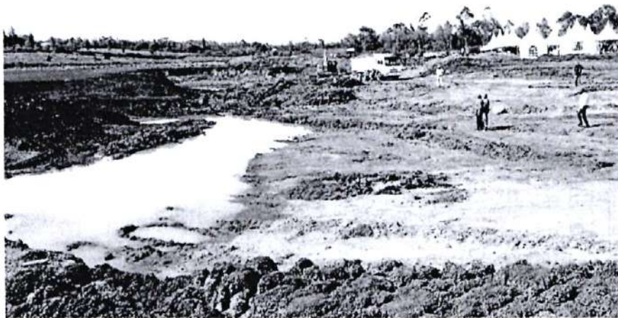
Ongoing construction works on Lusoi dam
