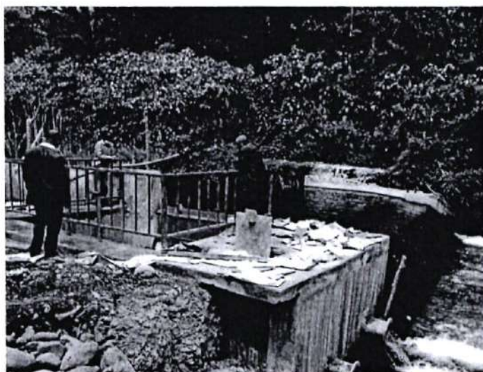
Mutoigu intake at Gura River
