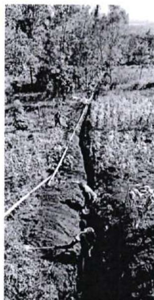
Construction of Simbara-Kamatongu Pipeline
