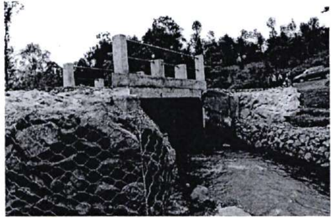
Riagitutu Bridge – Gikondi Ward
