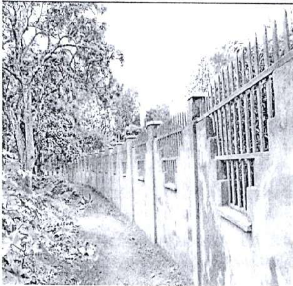
Perimeter wall at Ruring'u stadium
