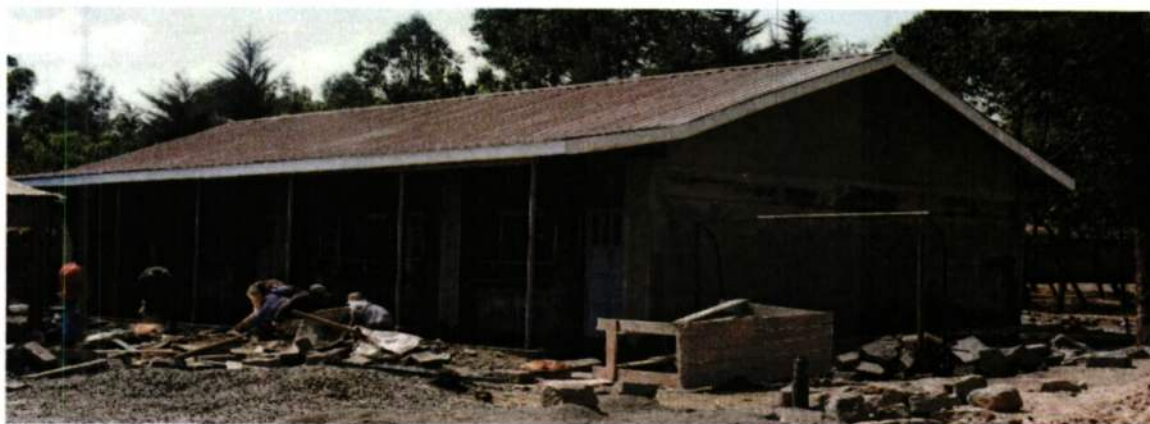
Classroom construction at Karundas ECDE in Thegu River Ward
