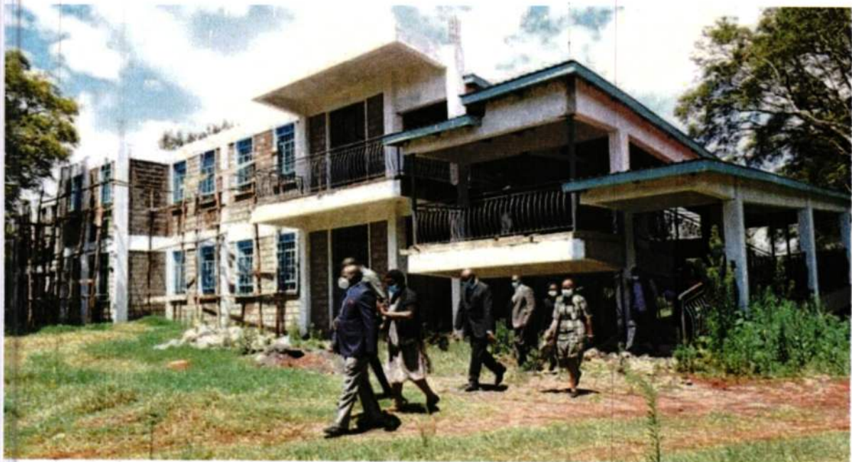
Construction of extension block at Mt. Kenya Hospital
