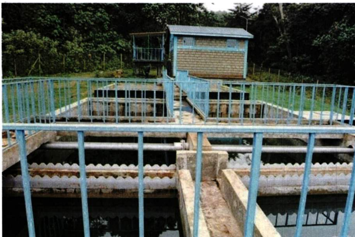
Narumoru water treatment project
