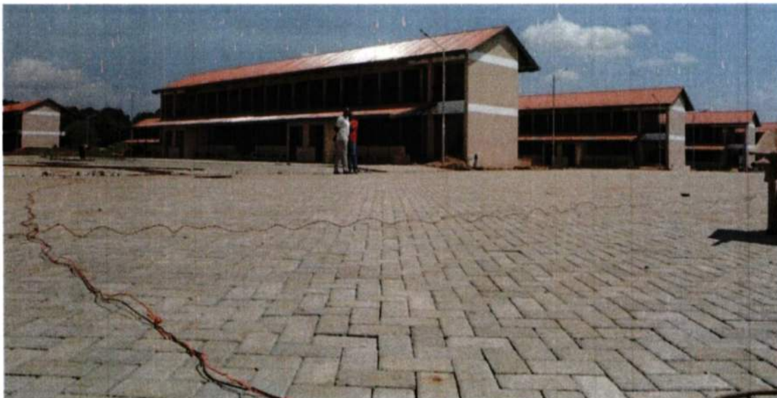
Upgrading and tarmacking of access roads to the Nyeri Town Bus Termini
