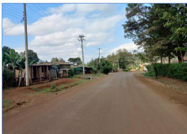
Tarmacked Road connecting the village areas
