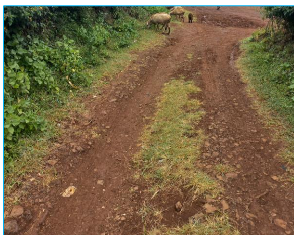
Narrow earth road
