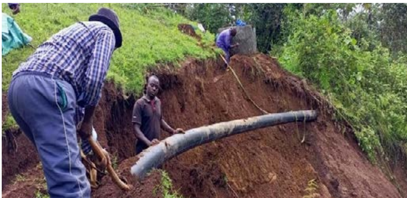
Figure 12: Community Members Anchoring a pipeline exposed by a landslide
