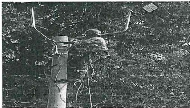
Installation of high mast street lights
